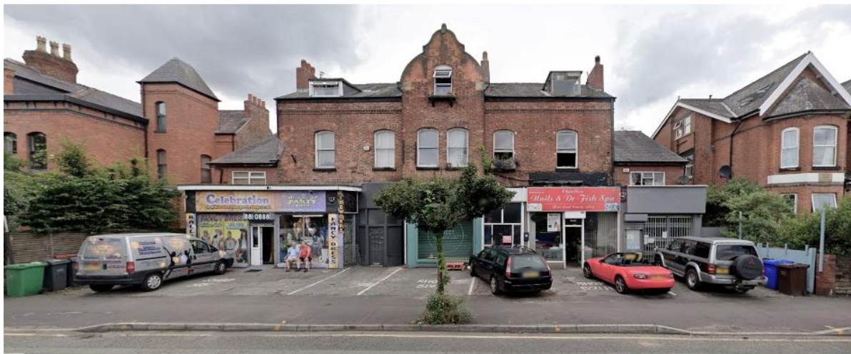
Front elevation from Barlow Moor Road
