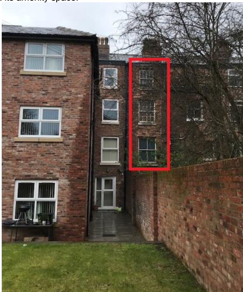
Rear of application property – the unauthorised extension is to the left - showing relationship with windows in adjoining 361 Wilmslow Road
