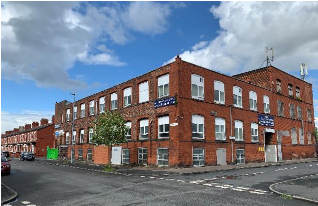
Photograph 2 View of the site looking North West from the corner of Crofton Street and Great Western Street
