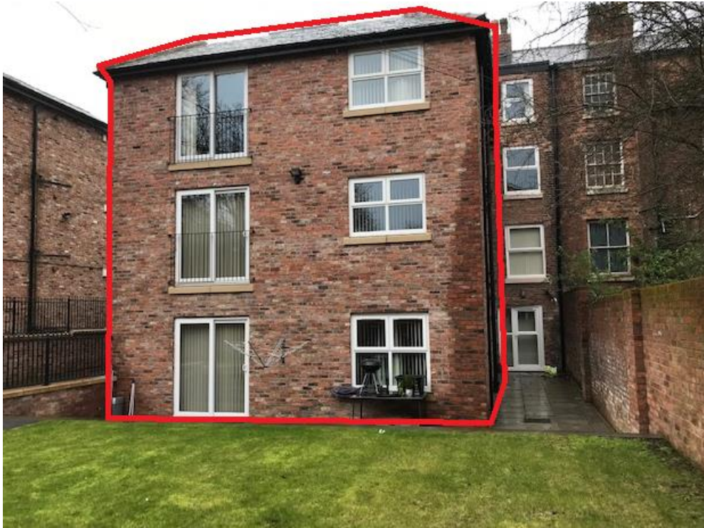
Unauthorised extension as viewed form rear of application property
