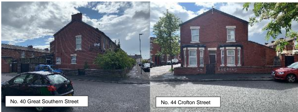
Photograph 6 and 7 40 Great Southern Street and 44 Crofton Street
