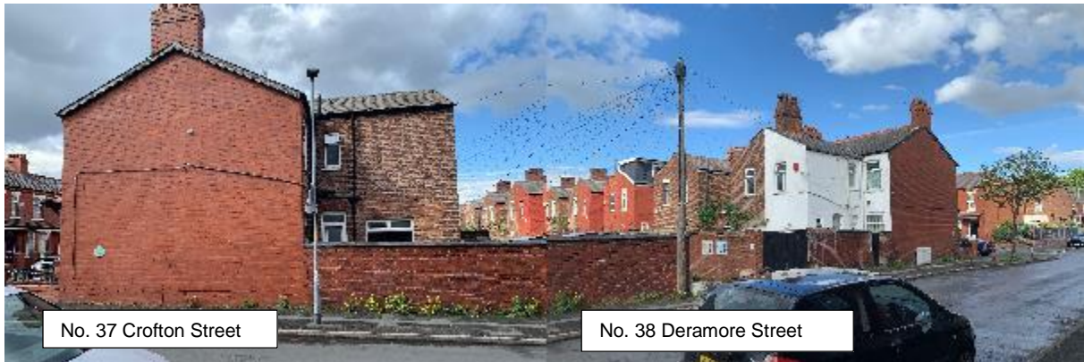
Photograph 4 and 5 No. 37 Crofton Street and No. 38 Deramore Street as viewed from the application site
